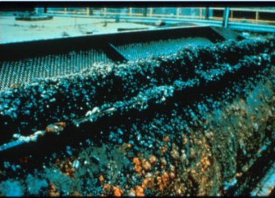
Encrusted debris screen
